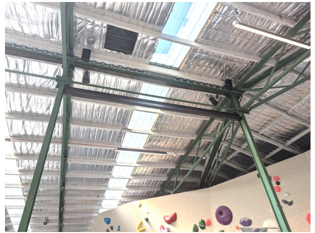
Once fitted, the new beam was painted to colour match the existing steelwork.
